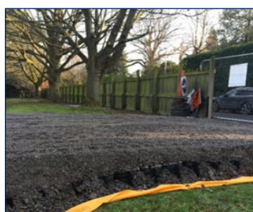
Geocell used for temp access
