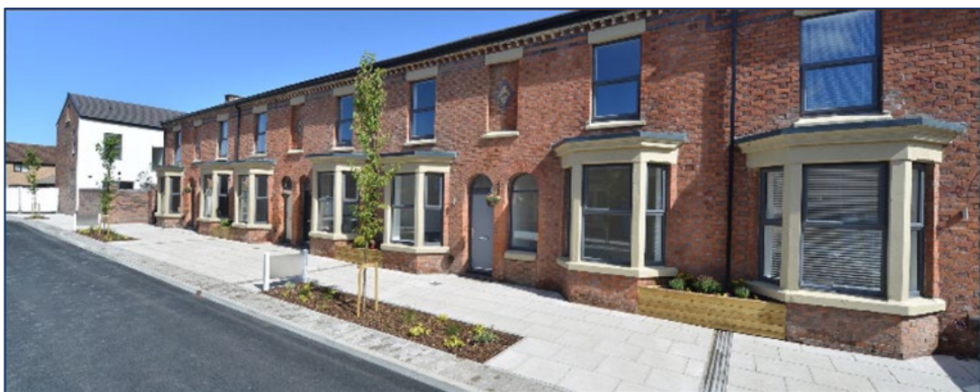
A new residential design – sustainable tree pits and sustainable raised planters utilised acting as street flooding intervention schemes
