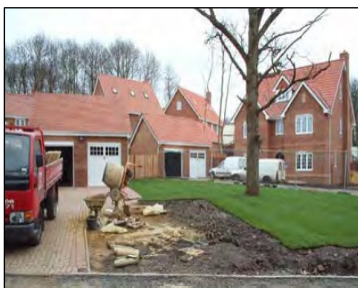
Roots not protected & compaction
