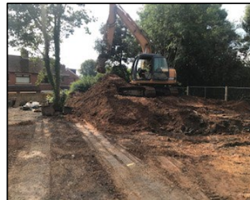
Material & machinery within RPAs – compaction
