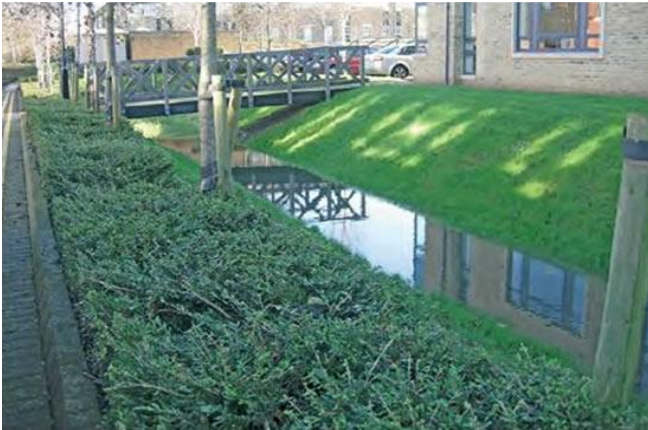
Rainwater harvest system
