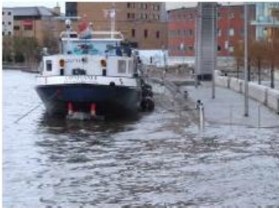
Figure 1: Photo of Belfast Lagside after a flood event
