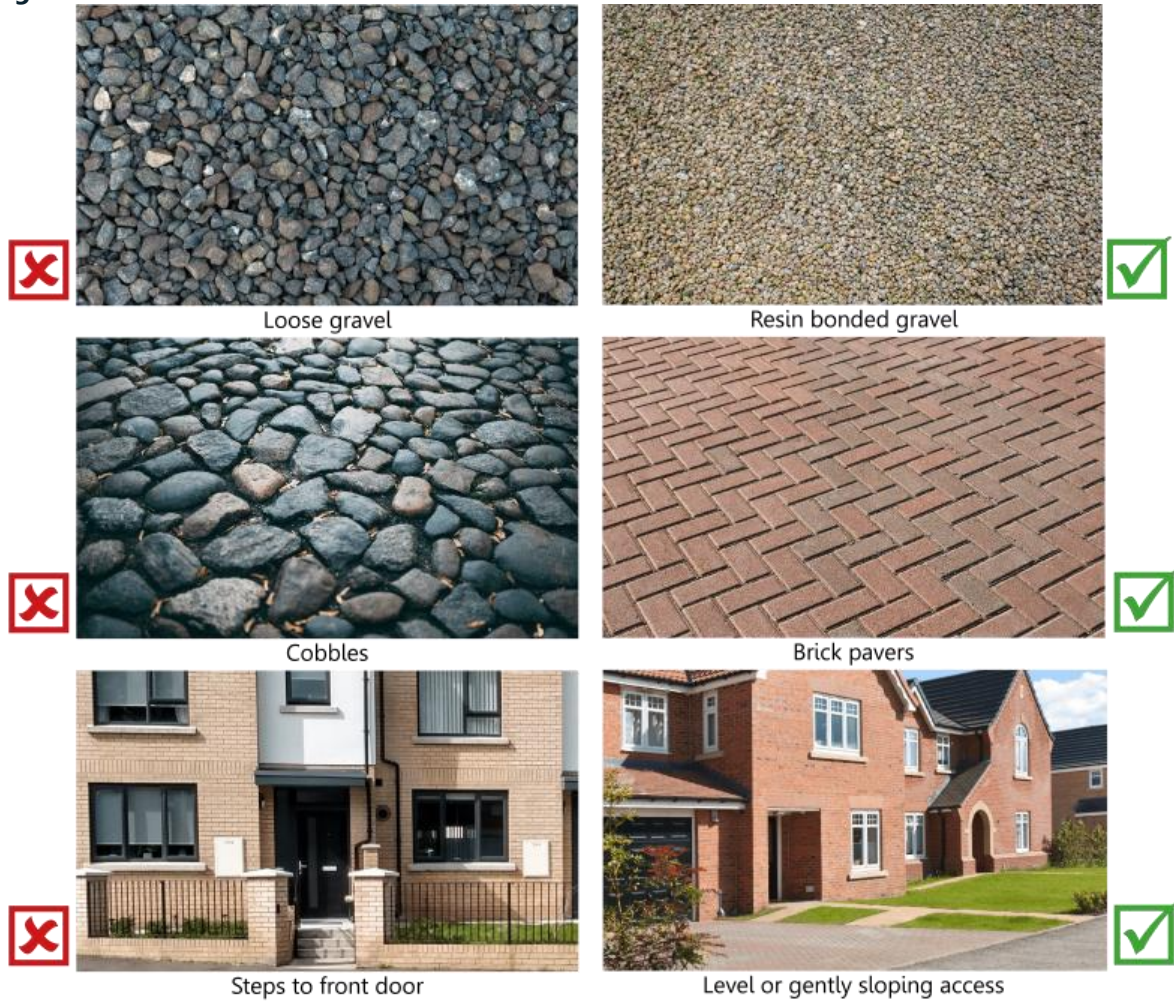
Figure 5.1: Accessible surfaces
