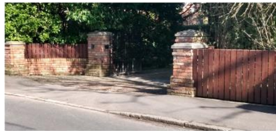
Mixture of brick and timber boundary treatment
