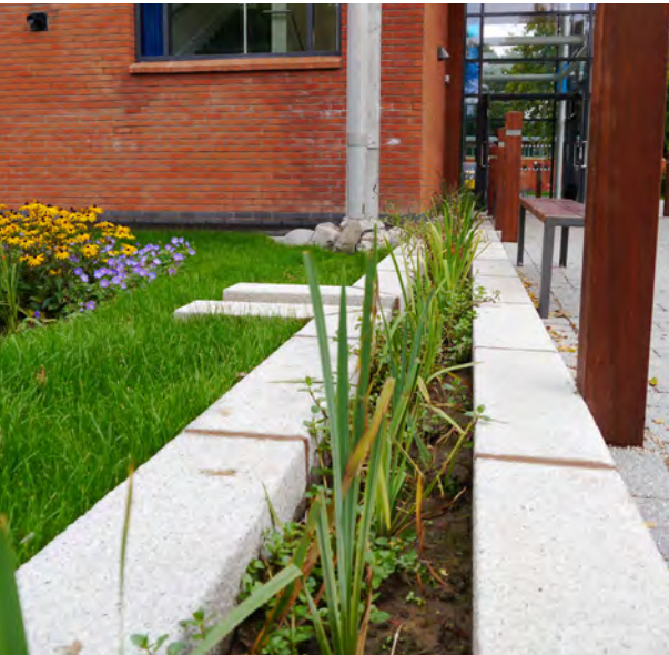
Wetland planted rill at Bewdley School.
