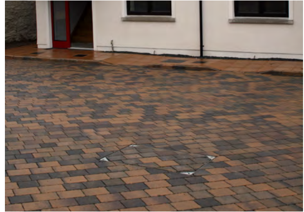
Permeable road in a housing development in Bangor.
