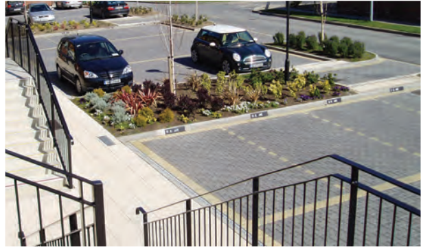
Permeable paving used in a residential car park.
