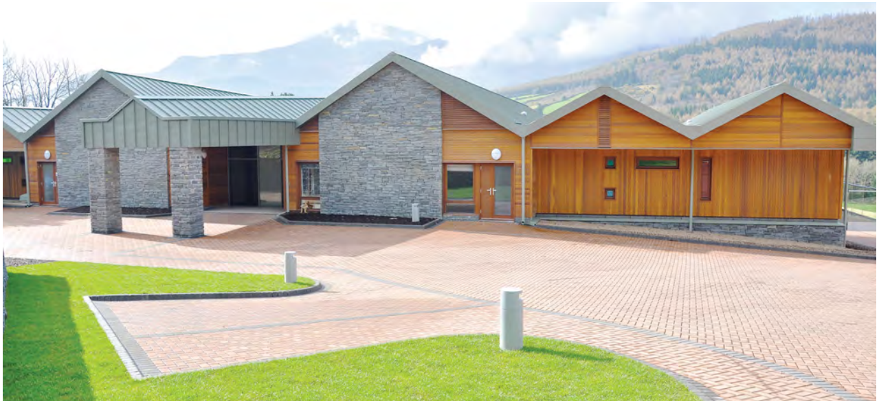
Fully infiltrating permeable pavement scheme at Daisy Hill Lodge, Newcastle.
