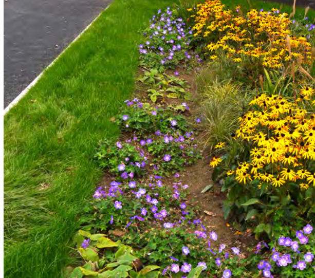
Filter strip between road and raingarden.
