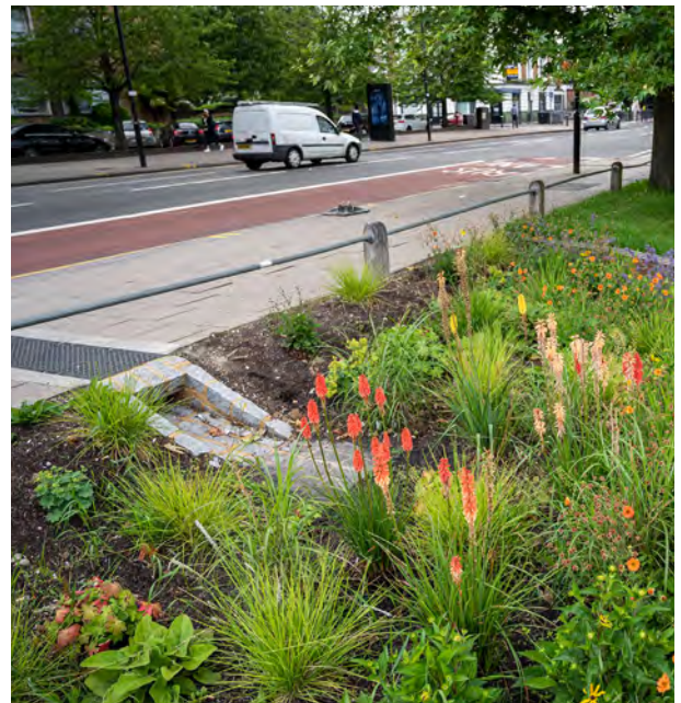
Raingarden at Crescent Gardens park.
