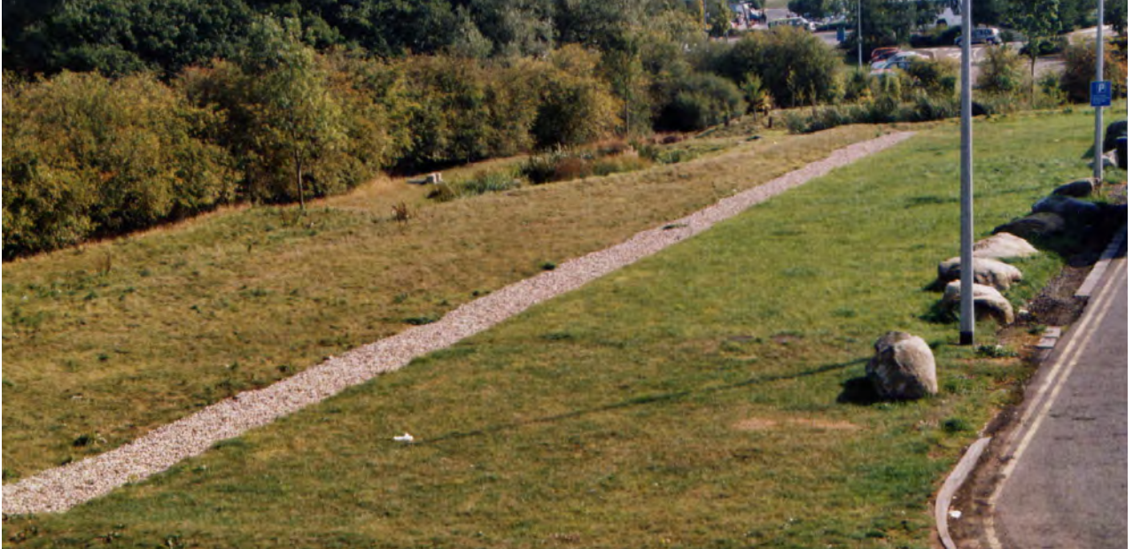
Filter drain beside a wide filter strip receiving runoff from a HGV parking area at Hopwood Motorway Services.
