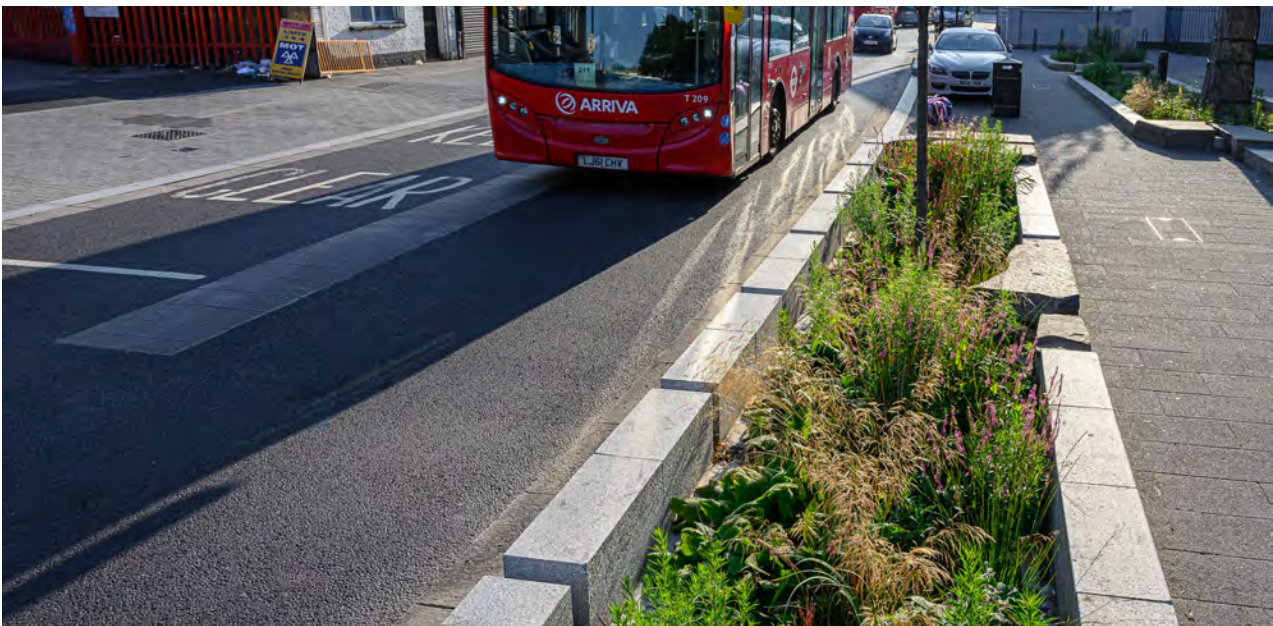
A bioretention raingarden receiving road runoff through breaks in the curb.
