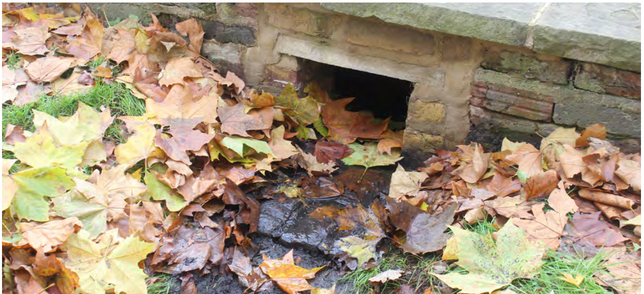
Polluted silts collecting at an inlet point from a busy road in London.
