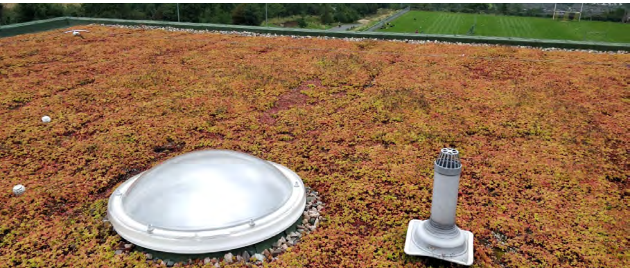
Recently constructed Green roof at a sports facility, Glengormley.
