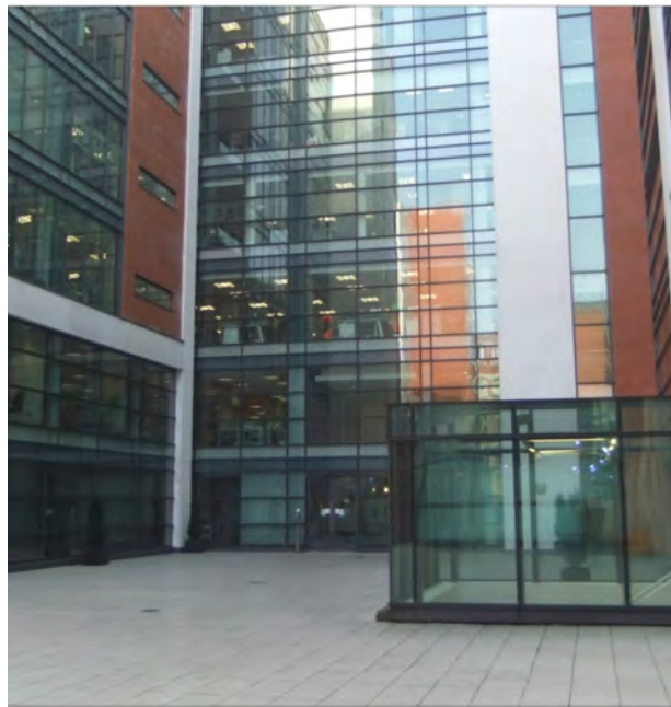
Courtyard using permeable pavement off Adelaide Street
