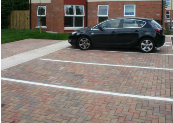
Permeable road in a housing development in Newtownabbey.
