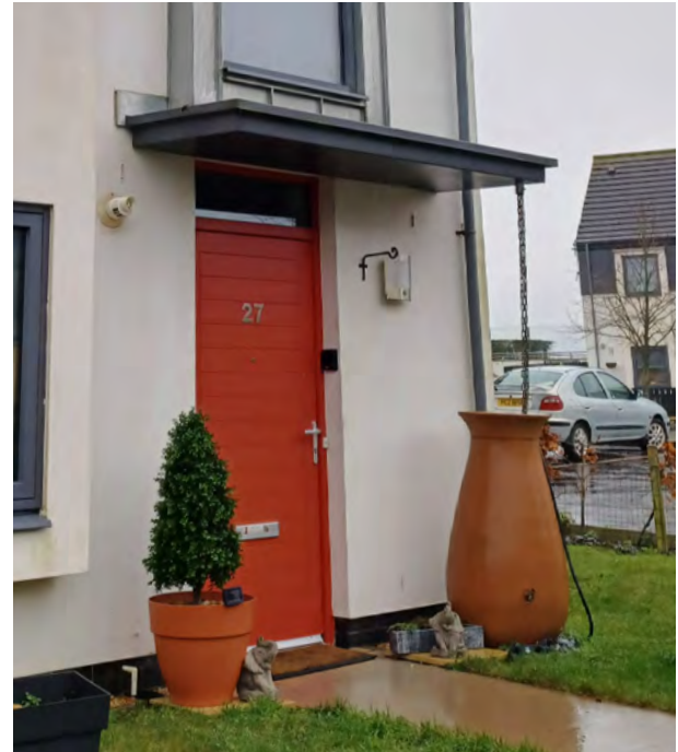
Use of a rainchain and modern rainwater butt, Carryduff.
