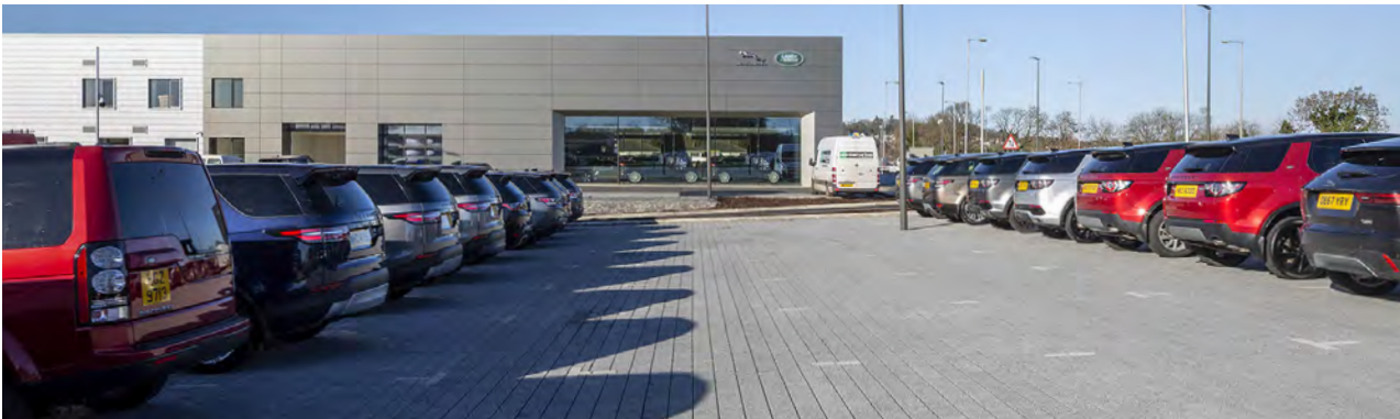
Permeable paving at a car dealership in Dungannon
