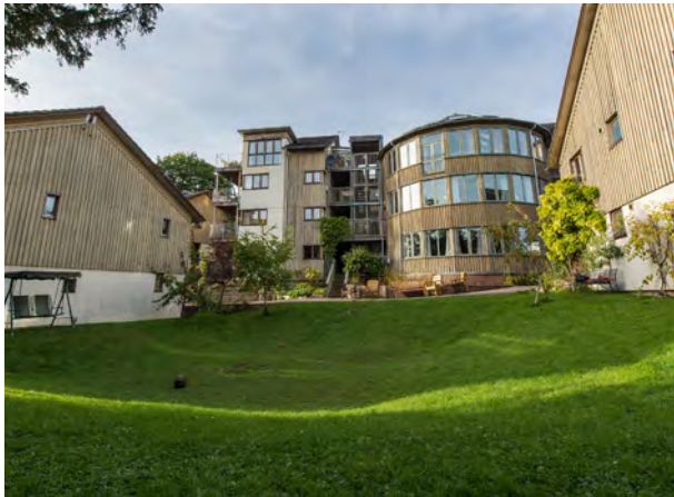
This play area at Springhill Co-housing also manages runoff - but only in extreme events.
