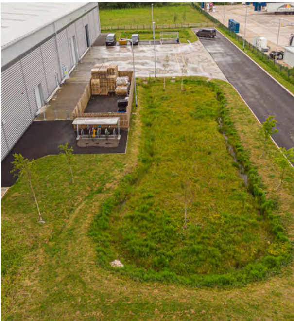
Meadow basin at Robert Welch warehouse.
