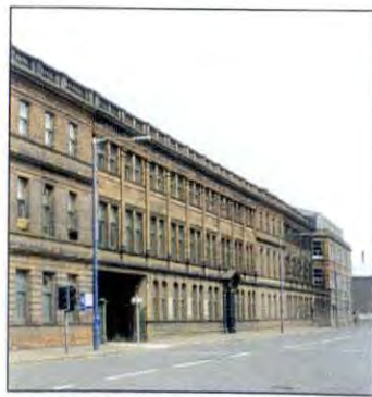
5. Former H & W HQ building
