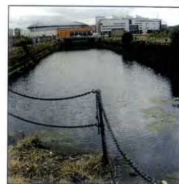
6. Hamilton Graving Dock
