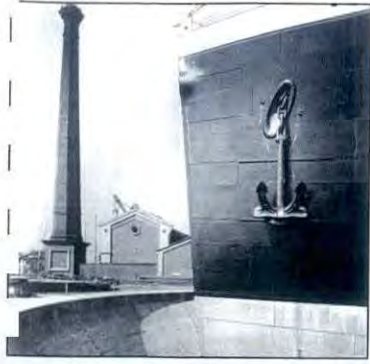
Thompson Graving Dock was specifically constructed for the fit out of the Titanic class vessels
