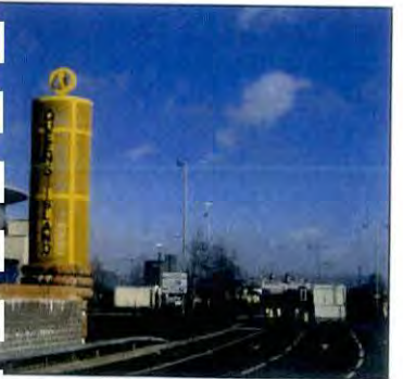
Existing access to Queens Island from M3
