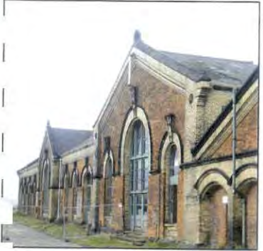
Thompson Dock Pump House
