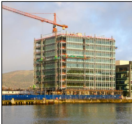
Figure 2.2: Construction of Grade A Offices at City Quays
