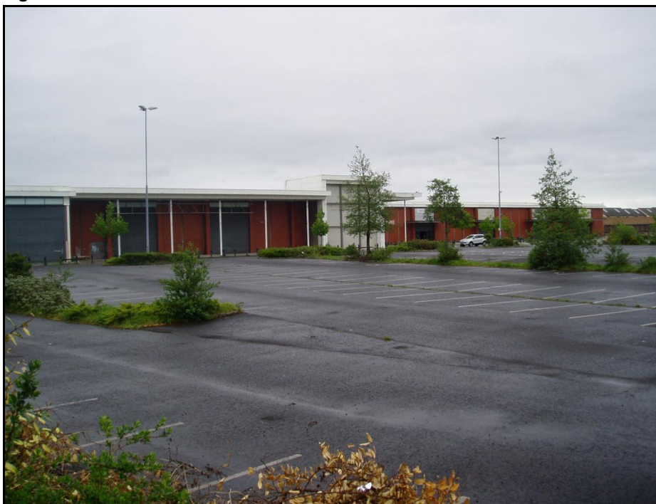
Figure 3.21: The vacant Hillview District Centre
