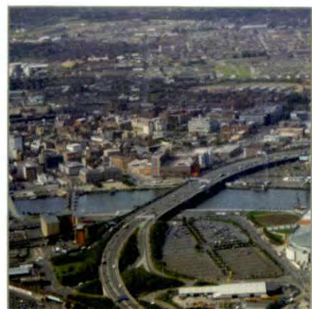
Aerial view over the M3
