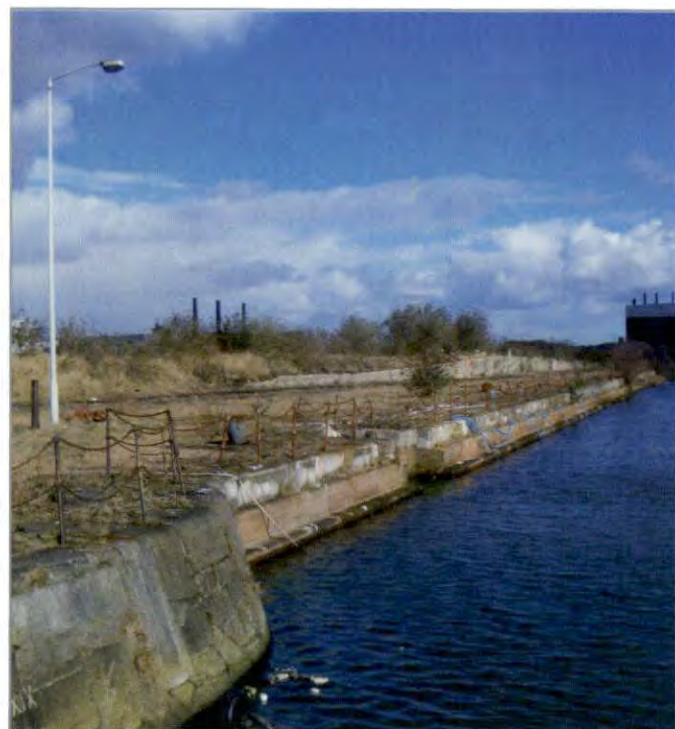
Current condition of Hamilton Dock
